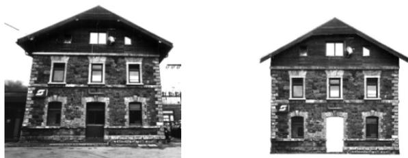
Fig. 3 An example of creating an orthophoto of a building. On the left — the original image of the building, on the right — an orthophoto
