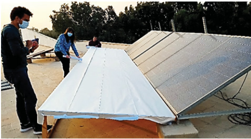
Fig.16 Fixing of the reflectors
