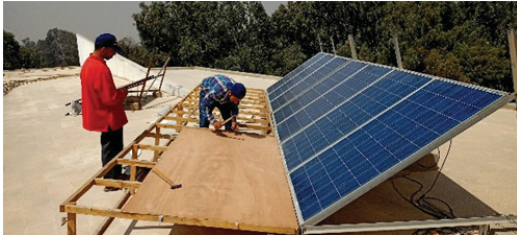
Fig.15 Covering the chassis by thin wood layer to attach the reflectors
