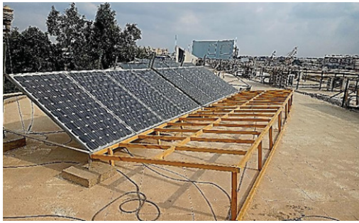
Fig.14 Building the wooden chassis of the reflectors
